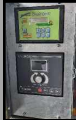
INTERFACCIA CON CENTRALINA IRRIGATORE E CONTROLLO GSM INTERFACE WITH IRRIGATION CONTROL UNIT AND GSM CONTROLLER
