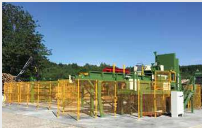
Safety barriers to delimitate the working area
